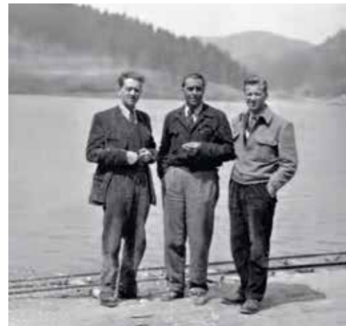
Vinodol HPP construction
