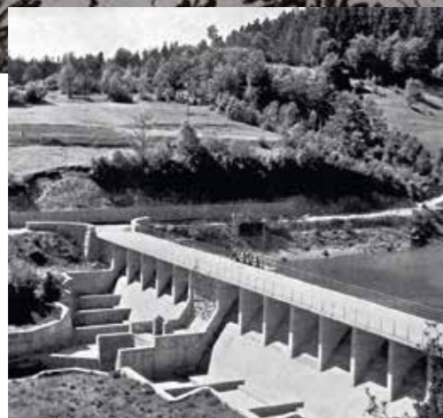
Vinodol HPP – Bajer Dam
